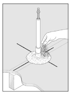
STEP 6: Using Play/Silica sand, cover the sealant. This step prevents debris from sticking to the sealant while drying and gives it a clean, finished appearance.
